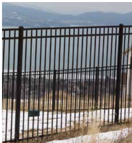
Above: A solid top rail and narrow vertical bars on this iron fence reduce hazards to wildlife.
