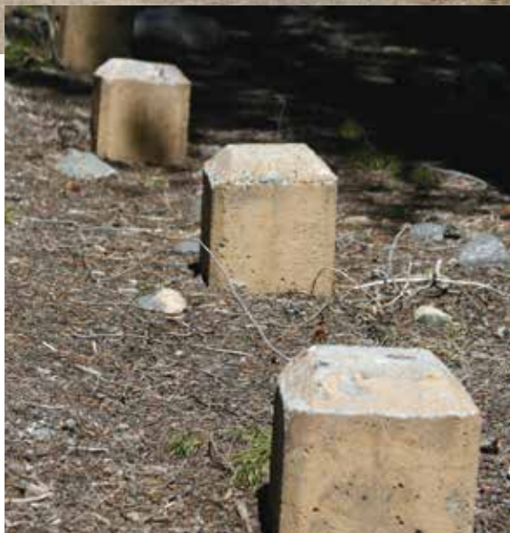
A row of boulders or bollards (concrete or wooden posts) can prevent vehicle access but pose no barrier to wildlife.
