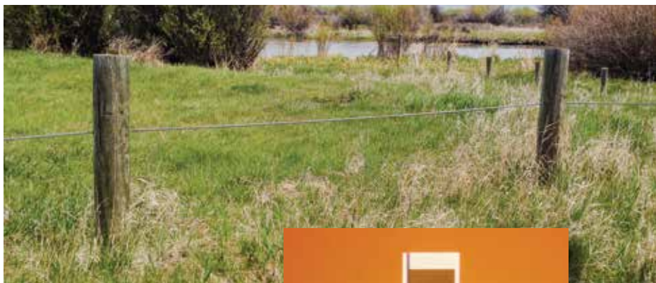
Above: A low post and single cable or chain fence creates little hazard to wildlife if it can be easily seen.
