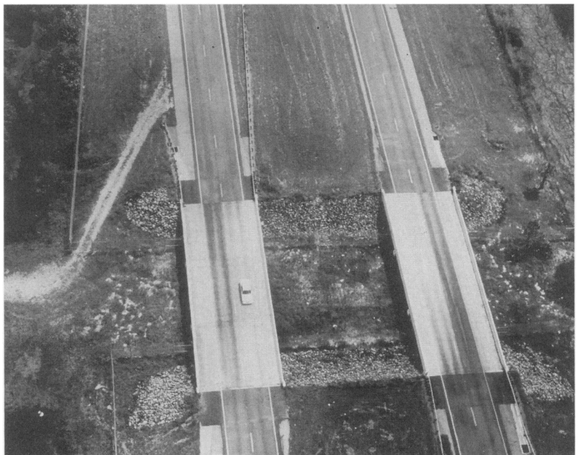
Fig. 2. Typical wildlife underpass and fencing at Interstate 75, southern Florida, 1992.
