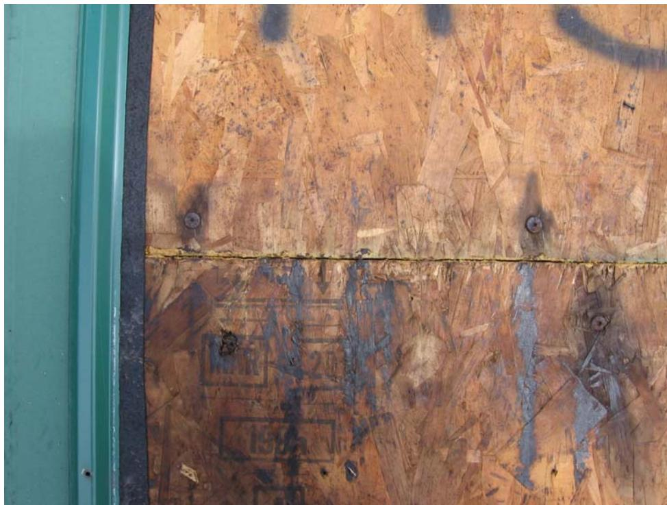
Photograph 2 – Fastener corrosion, blackened sheathing, and no spline or diaphragm nailing. Spray foam insulation visible in joint. Bottom left fastener sunk through the plywood.
