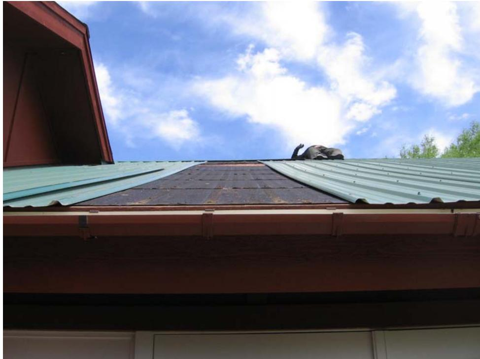
Photograph 1 – Area of removed roofing for inspection. Note visible sagging of the roofing.
