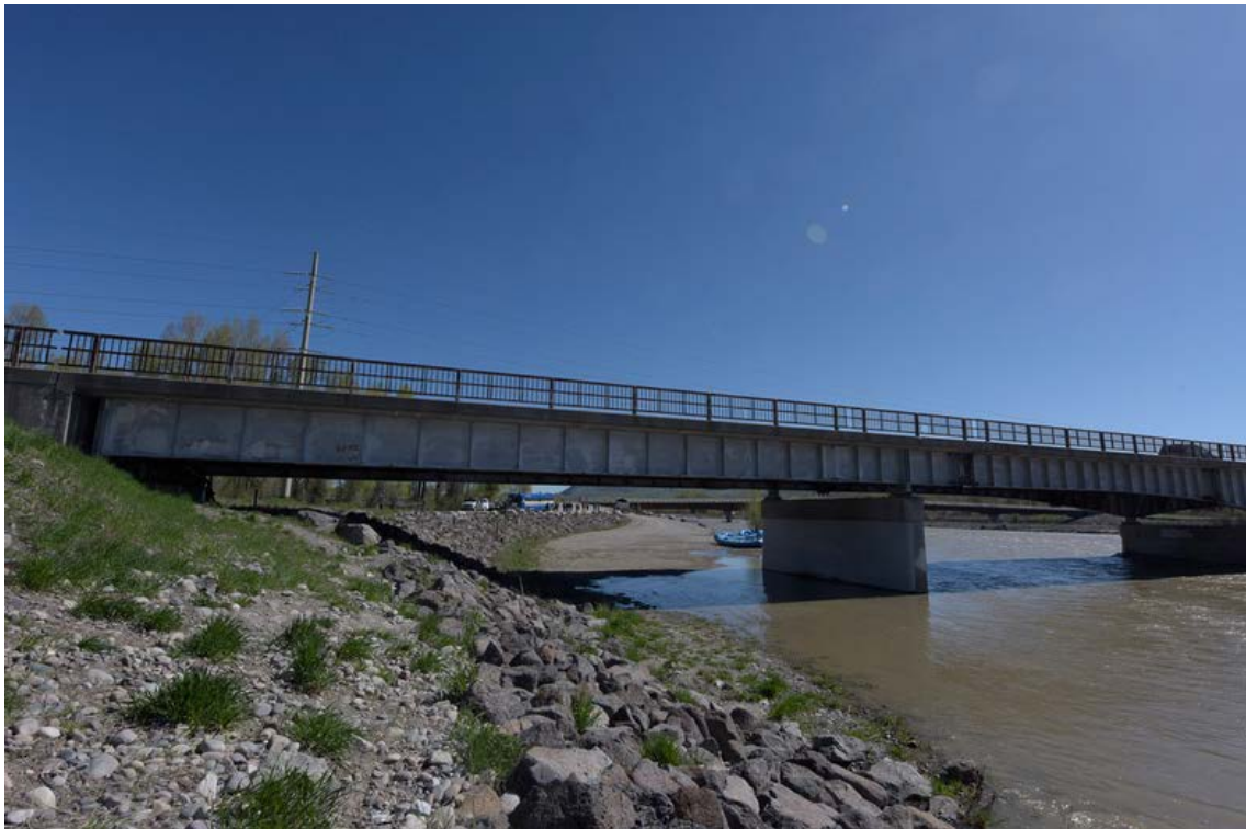
Figure 23. A bridge (WY 22, Snake River, west bank).
