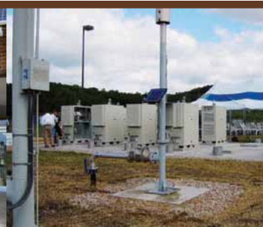
Microturbines at the Sauk County, Wisconsin, landfill.
